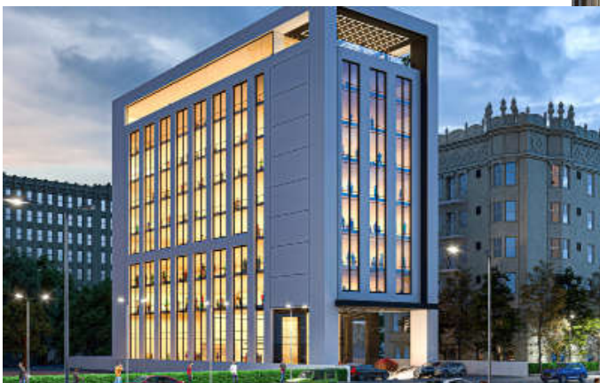
13 Storey, Commercial building, Hali road Gulberg-II, Lahore.
