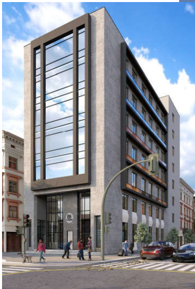
11 Storey, Commercial building, Shadman-II, Lahore
