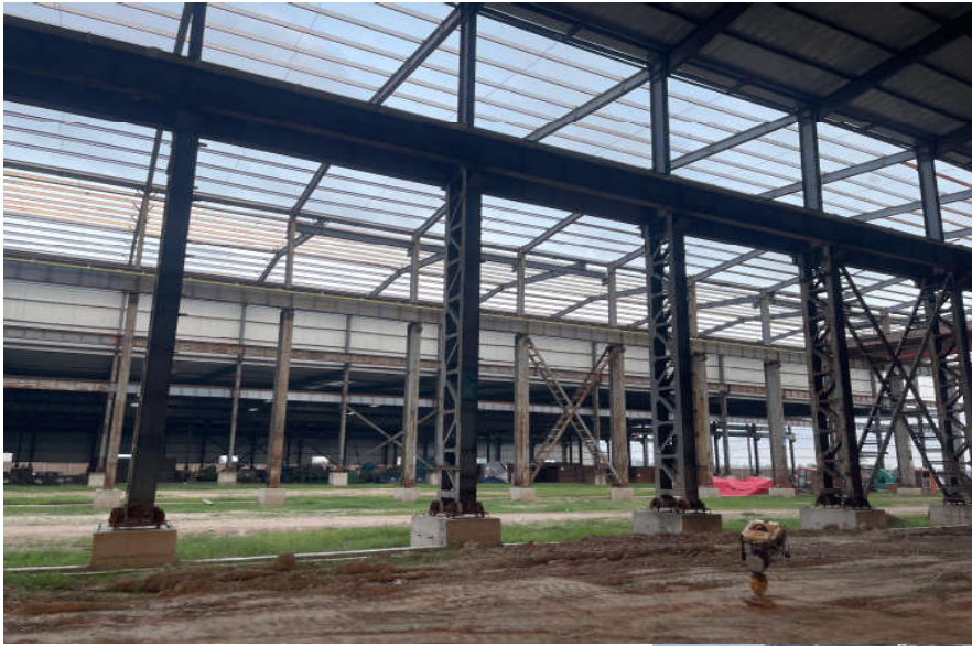
Forest Steel Faisalabad Multi-Bay Shed (Seven Sheds) Erection.
